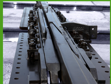
Manganese Three-Piece Bridge Joints (Swing Span)
