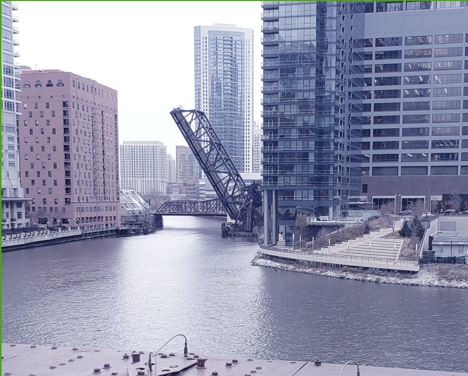
ATT Bridge Joint over Chicago River
