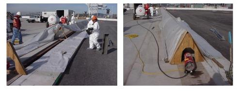
Hot Weather Grouting: [High temperatures accelerate set, decrease working time, and accelerate strength gain of epoxy products. The procedures below may compensate for these conditions.]
