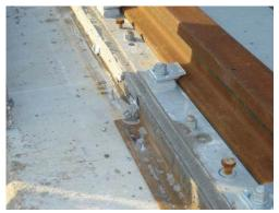
Placement: Grout must be placed without interruption. Should a delay occur beyond the working time of the material, all equipment used in mixing and placing the epoxy grout, shall be cleaned.
